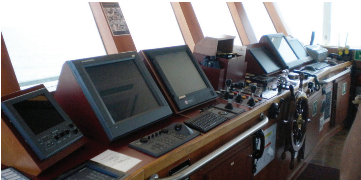
A view of the bridge
